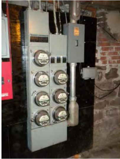
Electrical meters located in the basement
