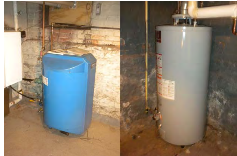
Typical indirect storage tank (left) and gas-fired water tank(right).
