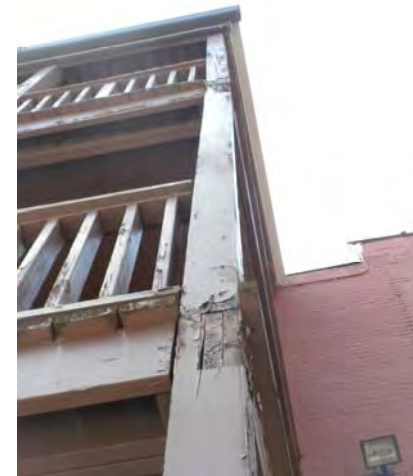
Wood damage and deterioration to an older deck structure
