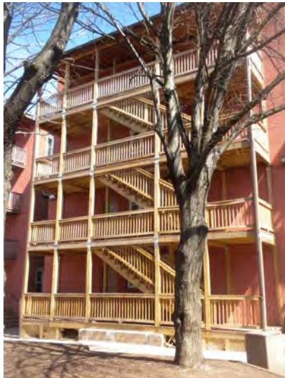
View of the recently rebuild rear deck structure
