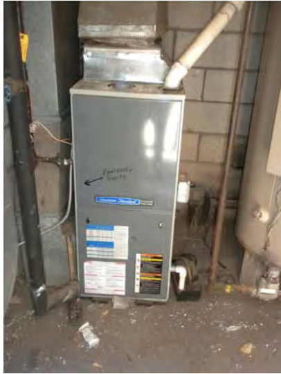
High efficiency furnace located at the community building
