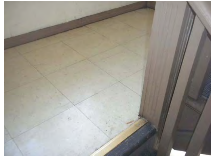
Typical VCT flooring in stairwells and hallways
