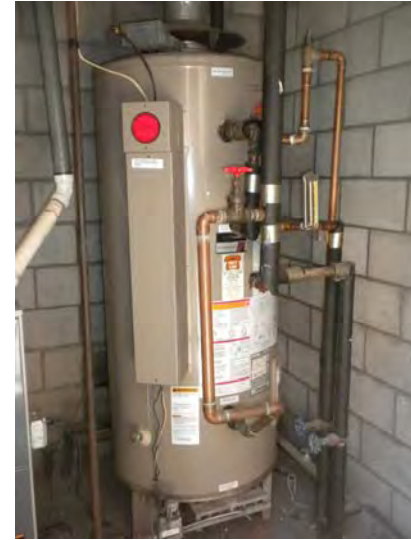
Laundry room domestic hot water tank
