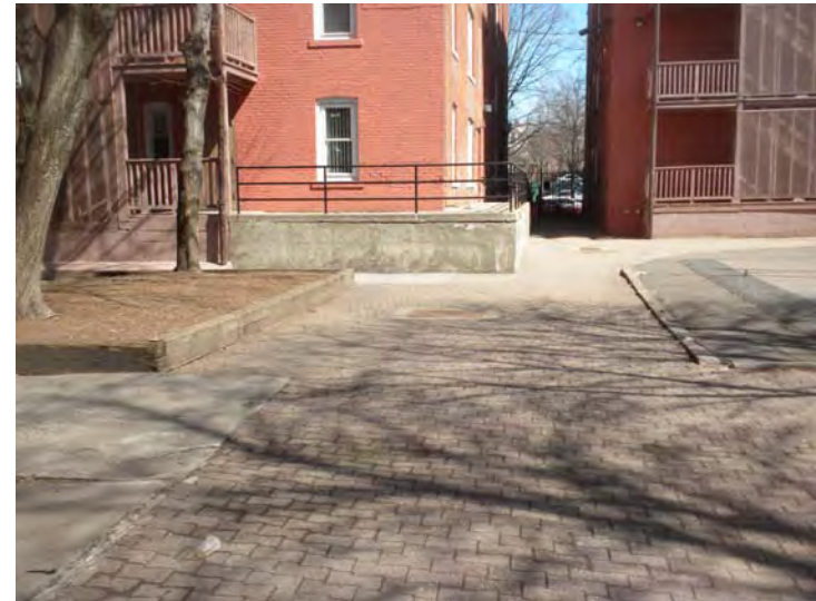
Partial view of the courtyard interior. Note the uneven brick and curb (trip hazards).
