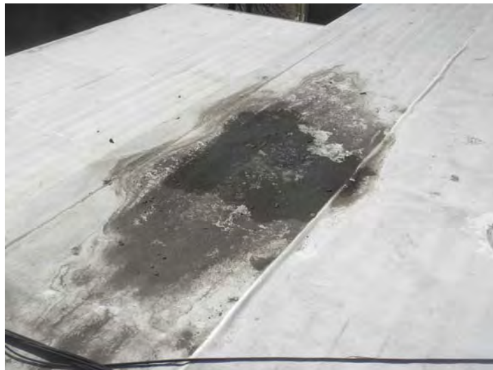
View of a recent leak at building one
