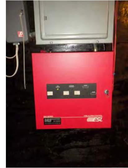
Typical fire alarm control panel
