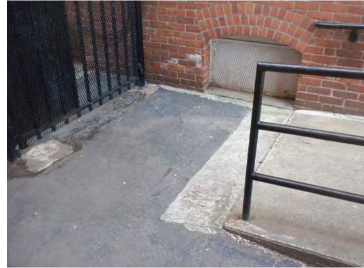
View of the non-compliant ramp landing and railing
